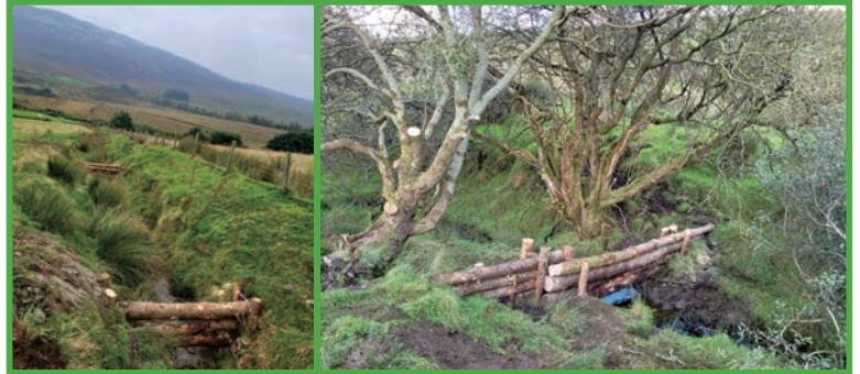
Natural Flood Management - delivery of Ireland's first leaky dam project.
