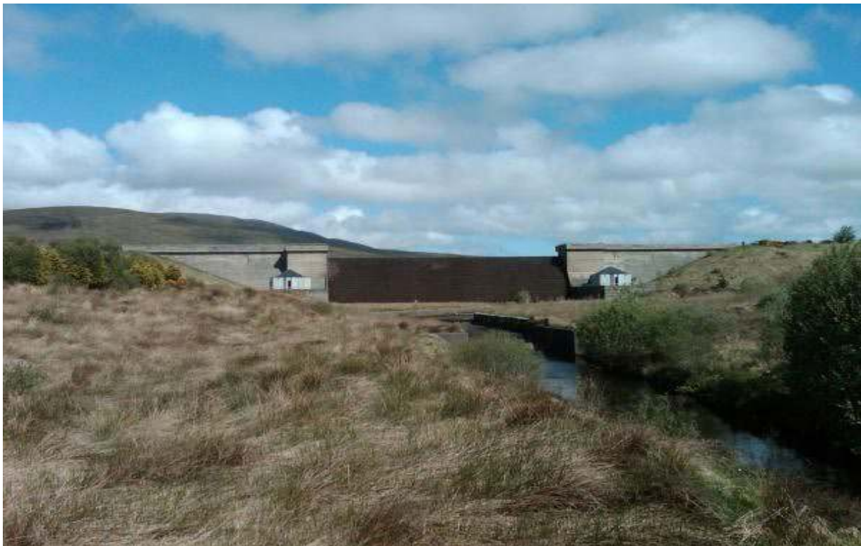
Figure 4.1: Eddie Fullerton Dam, Illies, Inishowen, County Donegal
