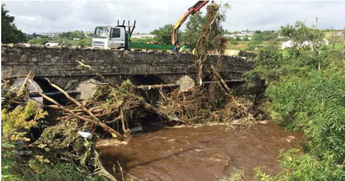
Figure 3.1: Example of the impact of the flood on 22 August 2017 and the large amount of woody debris that was ripped from the riparian corridors and accumulated at pinch points such as the Cockhill Bridge in Bunrana.
