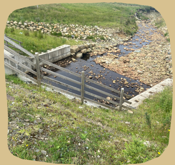
Barriers on streams prevent sediment transport and are barrier to fish movement
