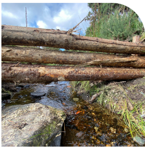
A log leaky dam on the Bocharney River
