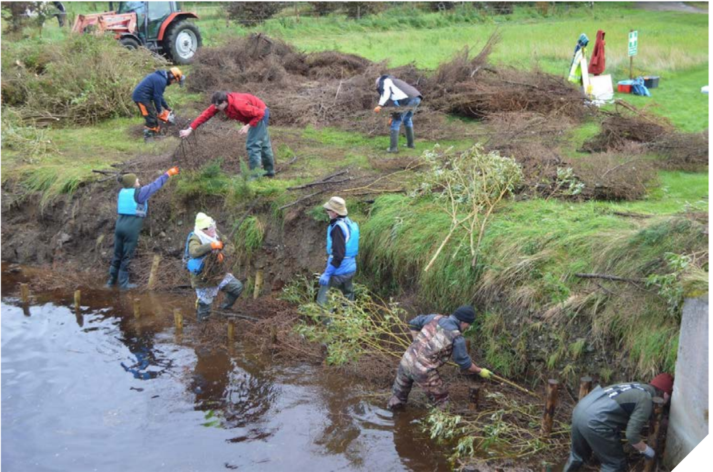
Natural bank revetment as part of the Glennagannon river restoration project.
