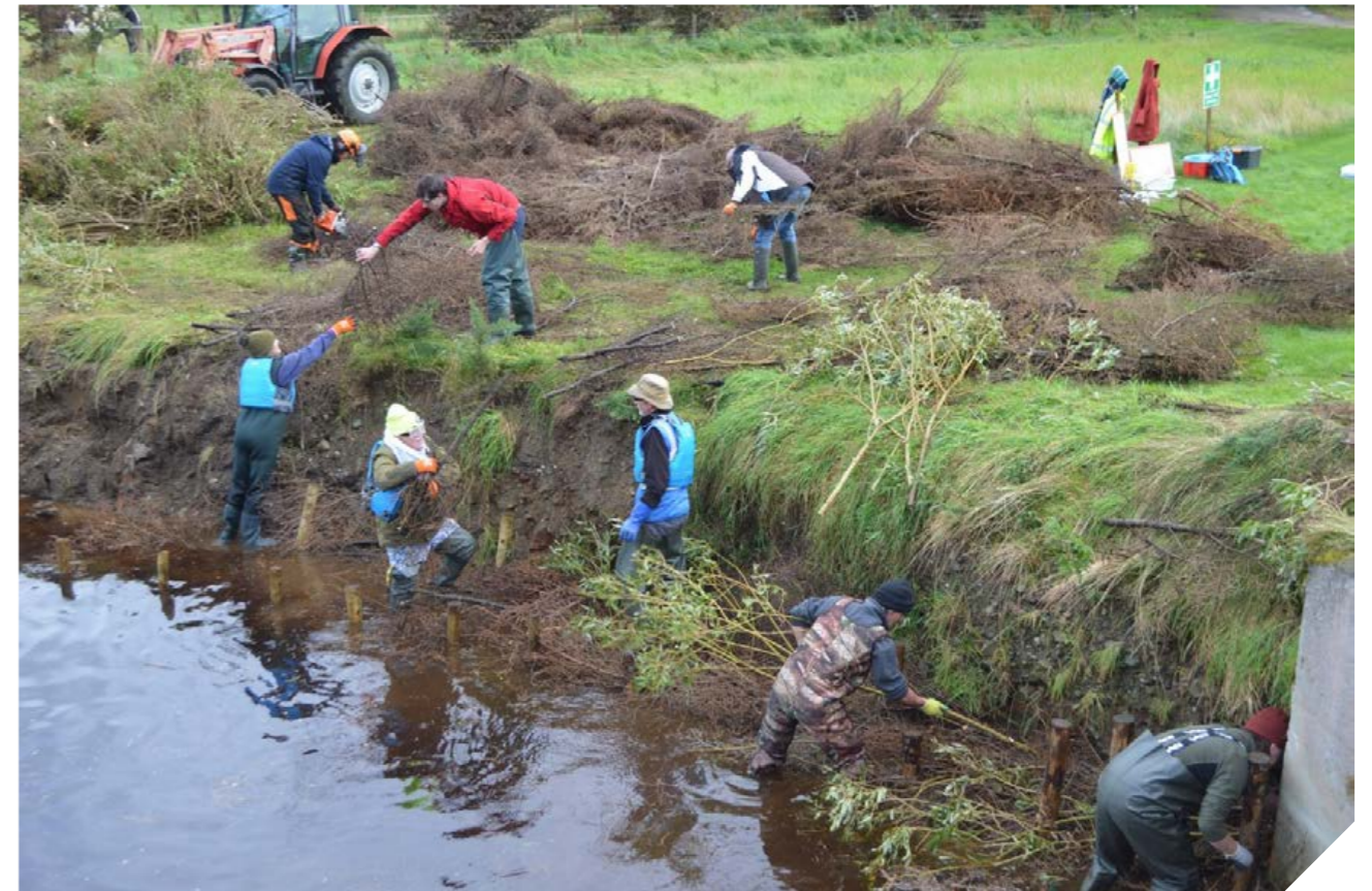
Natural bank revetment as part of the Glennagannon river restoration project.
